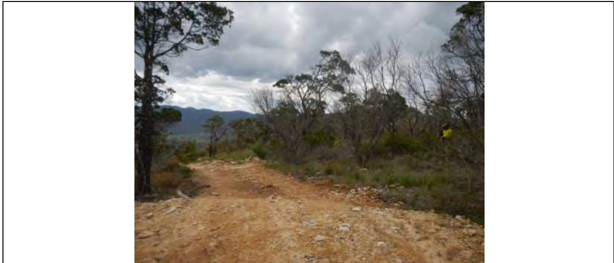
Plate 8 Recently cleared track 3.5 m wide close to ridge country on western boundary of site. Track is estimated to have been cleared in 2012. Person on right of picture is standing 10 m from left-hand side of track, which represents the proposed clearing width of tracks between turbines.
