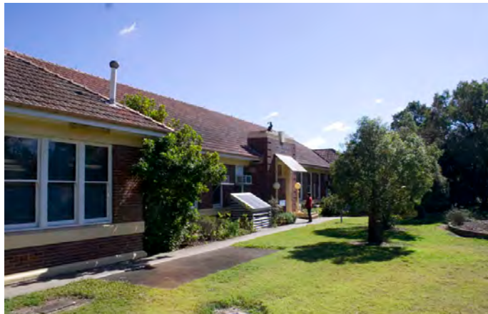
Veterinary School Main Building (heritage building)
