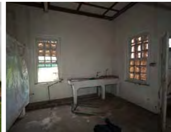
Animal Morgue interior with benches and other fittings intact
