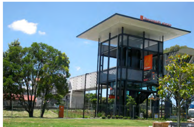
Pedestrian bridge over Fairfield Road to Yeerongpilly railway station
