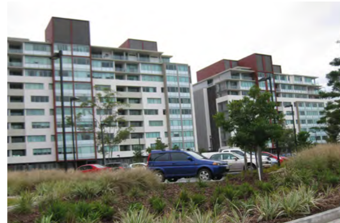
View north-east to Tennyson Reach apartments
