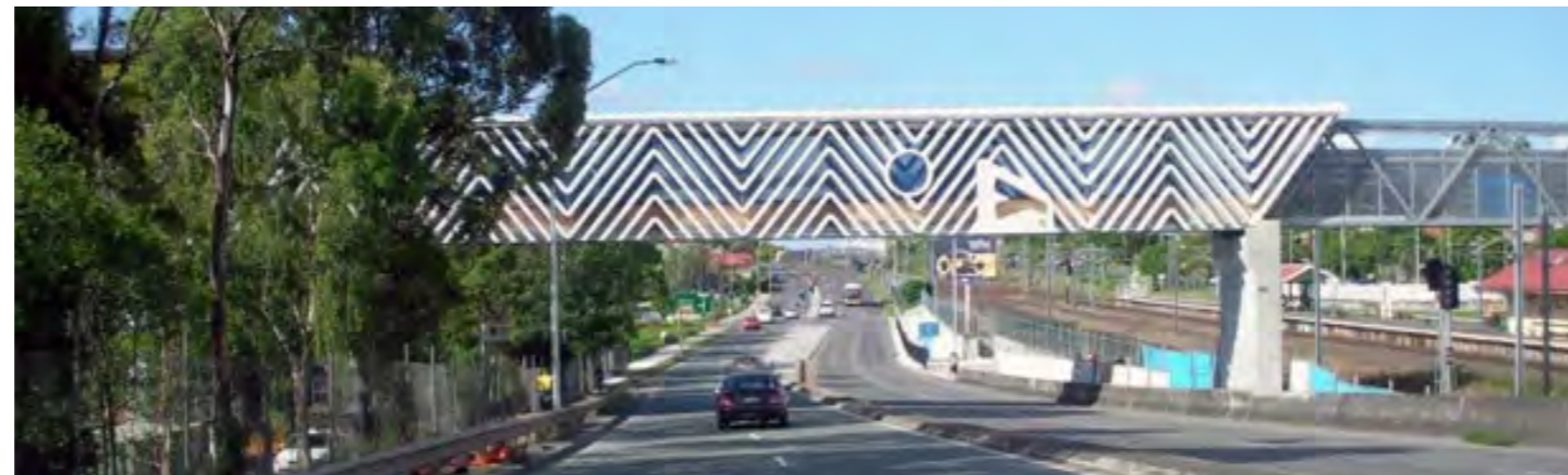
View along Fairfield Road travelling north with Yeerongpilly railway station to the right
