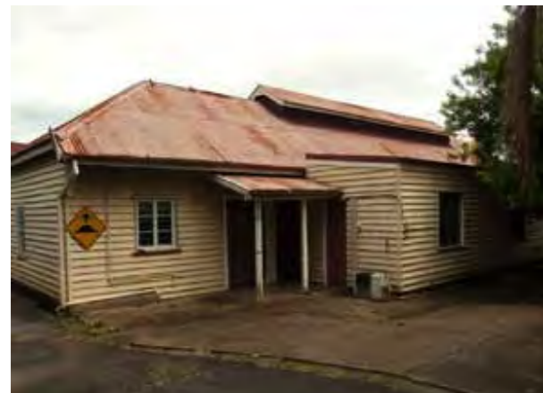
South-eastern corner of the Stables with skillion extension
